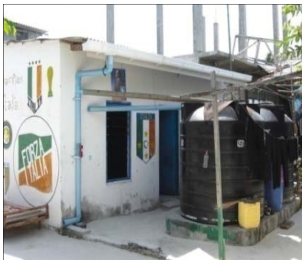
Photo 1. RWH System in the Maldives.
