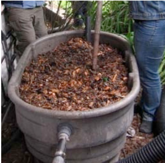
Figure 3.15: Mulch basin grease trap
