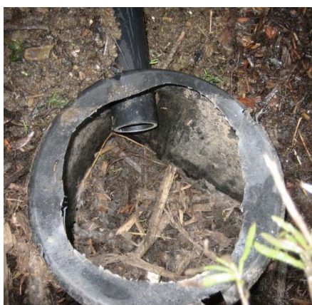
Left: A simple and cheap way to protect the greywater pipe from clogging by the mulch, it also permits to clean on a regular basis the accumulation of solids in that small perimeter of mulch.
