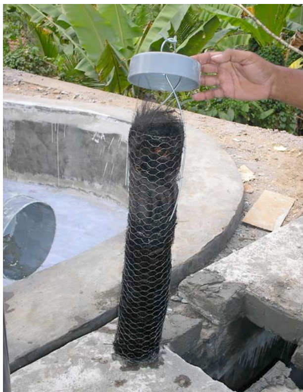
Figure 3.21: Handmade Filter with Ijuk
