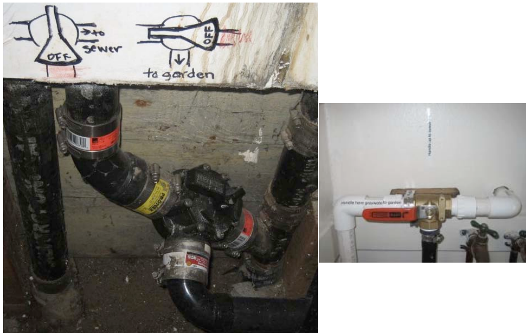
Figure 3.12: Examples of 3-way valve installations Courtesy: http://greywateraction.org
