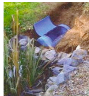
Figure 3.17: An example of a hand-made grease trap Courtesy: Campus Center for Appropriate Technologies (CCAT) http://www.appropedia.org
