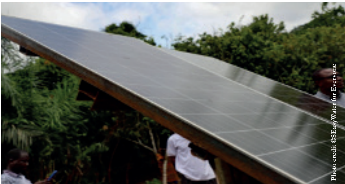
Upgrade of Water Station to Solar-Powered System at Monkrate Community – Dambai
