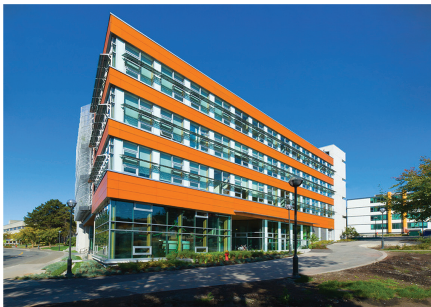
The University of British Columbia Centre for Interactive Research in Sustainability (CIRS) building in Vancouver (completed in 2011), uses a “Solar Aquatics System” – designed to mimic the purification processes of naturally occurring water systems in close proximity to human inhabitation, such as streams and wetlands. Photo: Don Erhardt, courtesy of University of British Columbia.
