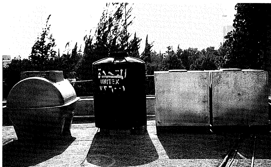
The four household storage tanks used in the study were made of (from left) fiberglass, polyethylene, and cast iron.
