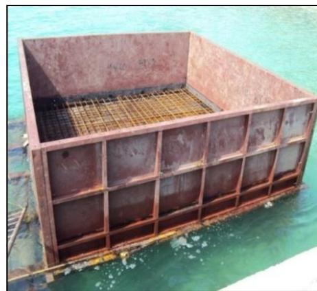
Fig. 32 Assembled steel caisson for P12 and 13
