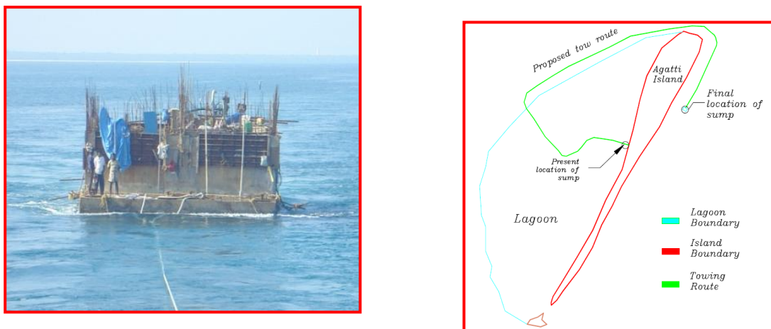
Fig. 9 Views of Sump during its Tow (left) and the towing route of Sump (right)
