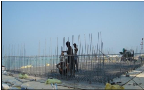
Fig. 22 Bed preparations for sump at lagoon beach
