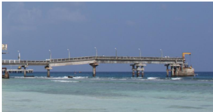
Fig. 45 View of the plate girder after completion
