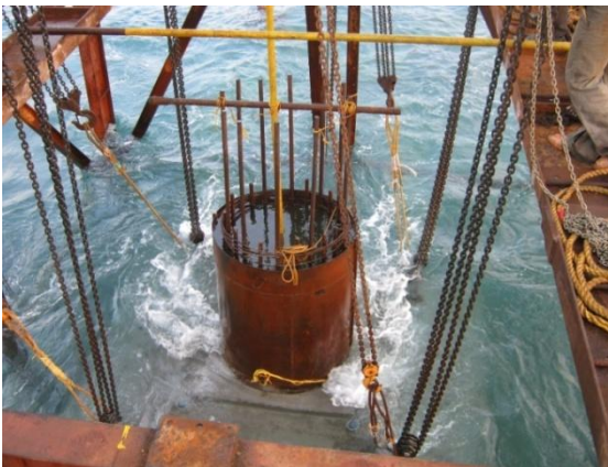
Fig. 38 Footing of P12 lowered in water
