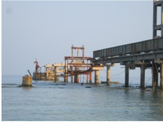
Fig. 40 Assembled plate girder on the bridge
