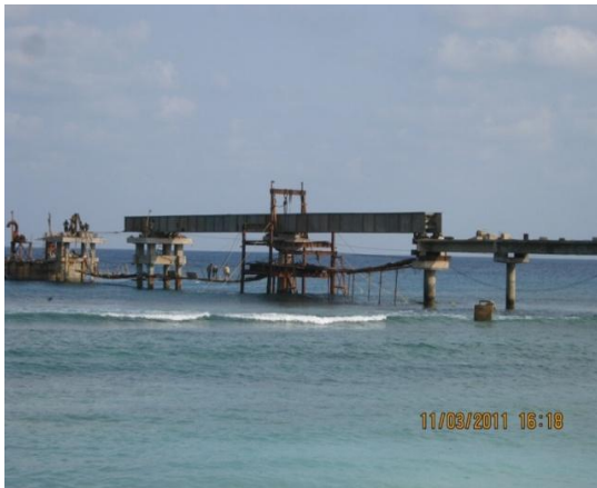
Fig. 42 Launching of plate girder
