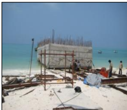
Fig. 24 Sump after pushing in to lagoon
