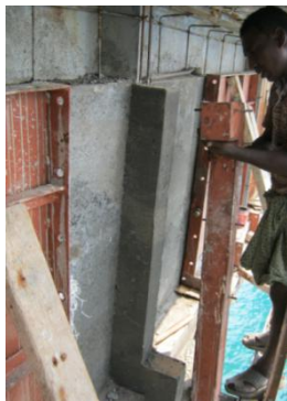
Fig. 44 Micro concreting work
