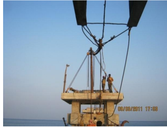
Fig. 41 Derrick for plate girder launching
