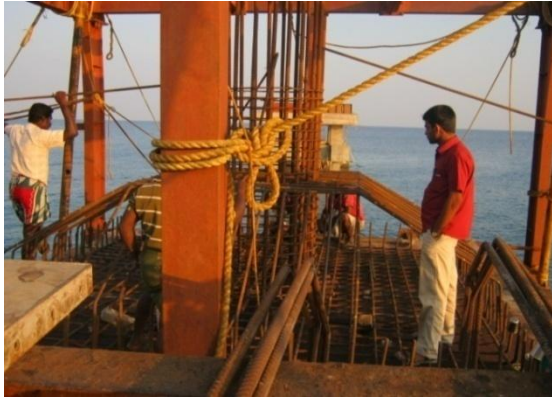
Fig. 36 Reinforcement work for P12 footing on stage
