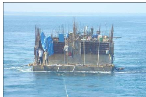
Fig. 27 Towing of Sump in open ocean at Minicoy
