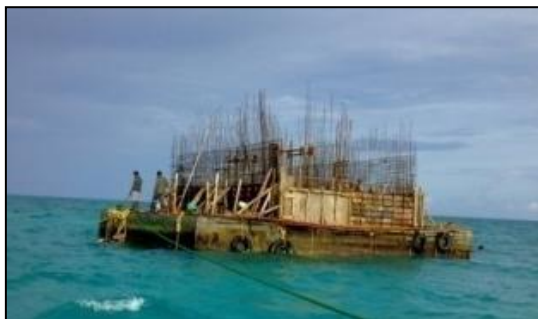
Fig. 26 Towing of Sump in open ocean at Agatti
