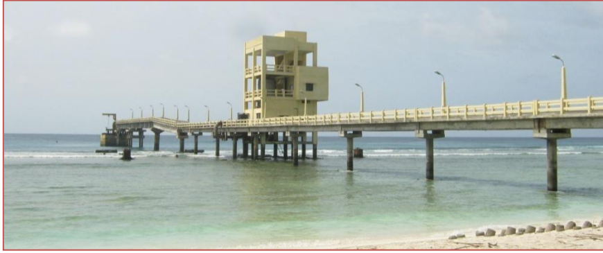
Fig. 10 Views of Agatti Plant showing the Plant Building, Bridge and the Sump
