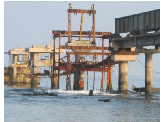
Fig. 39 Completed Section of P12 with pier cap
