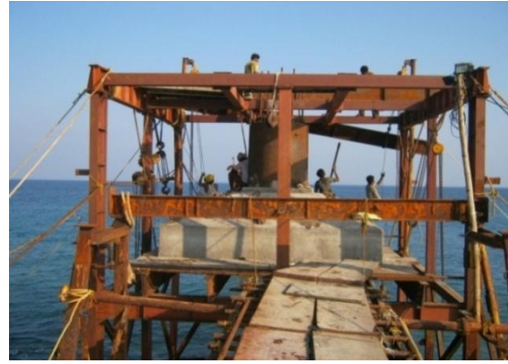
Fig. 37 Concreting work of P12 on steel stage
