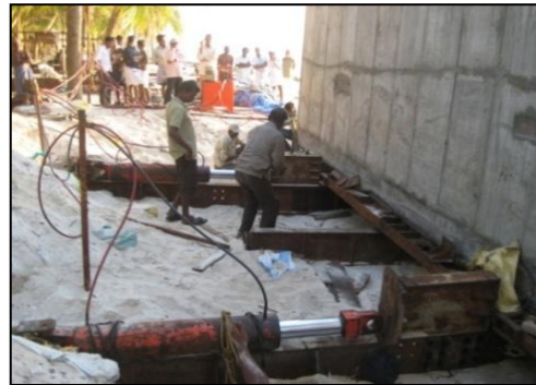
Fig. 23 Hydraulic jack for pushing sump
