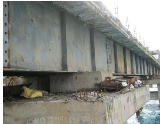
Fig. 43 Plate girder welded with bearing blocks
