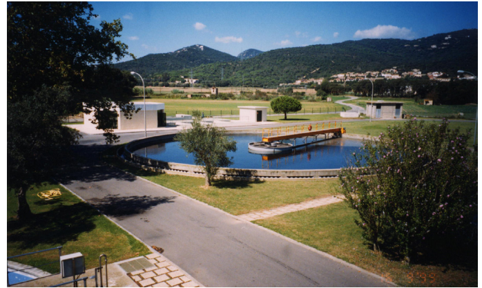
Figure 4. Castell - Platja d'Aro WWTP.
