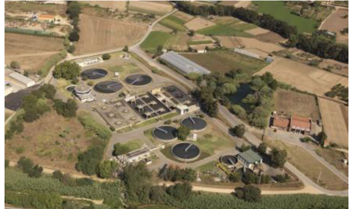
Figure 8. Castell - Platja d'Aro WWTP. Aerial view.
