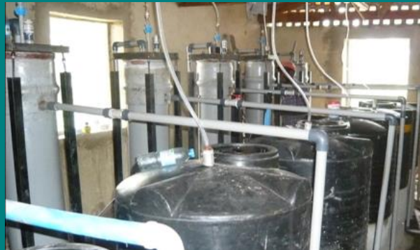
Six ClariWash filters installed in Western Uganda
