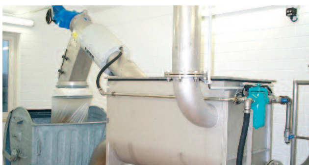
Tank-mounted ROTAMAT® Rotary Drum Fine Screen ...
