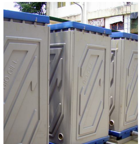
BioGill bioreactors were retrofitted to an existing STP in Manila to improve BOD reduction and reduce energy consumption.
