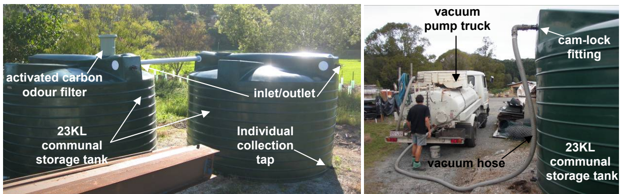
Figure 4: Communal storage tanks showing activated carbon filter and shared pipe (left) and vacuum pump out truck transferring the urine solution to a communal storage tank (right).
