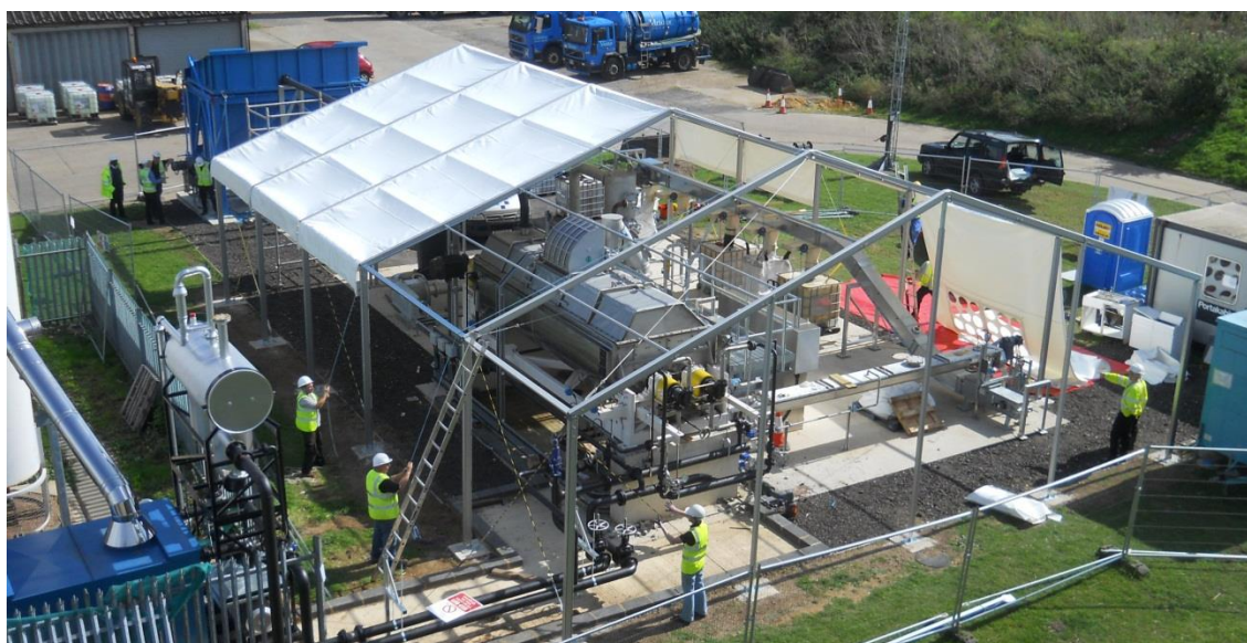
Figure 52 - Slough Dryer under Construction
