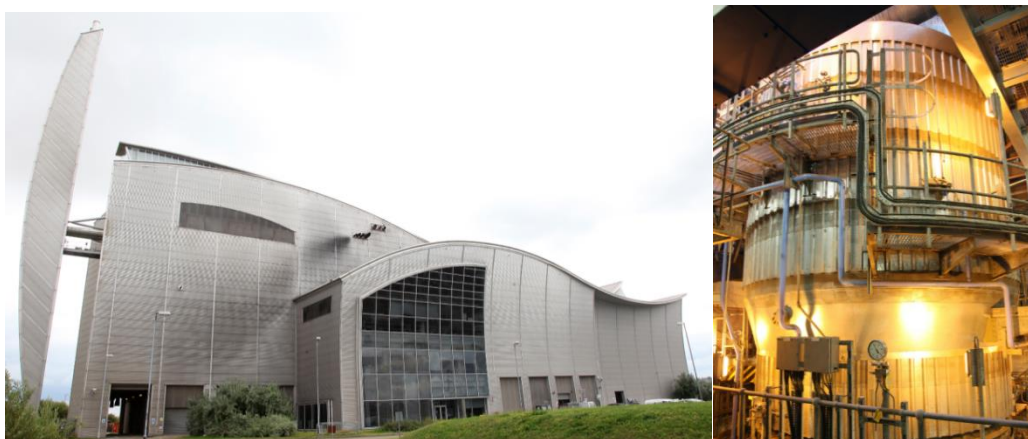
Figure 55 - left - Crossness SPG, right - 1 of 2 Fluidised Bed Incinerators
