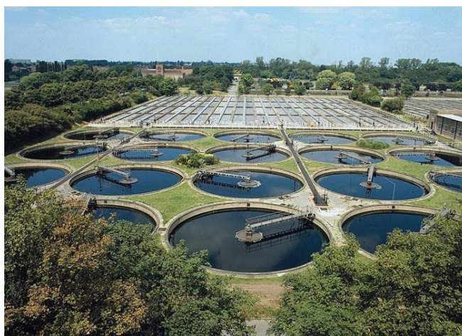
Figure 9 – Picture of Mogden STW showing the final Settlement Tanks in the fore ground with Aeration Basins visible in the background (TWUL-i 2011)
