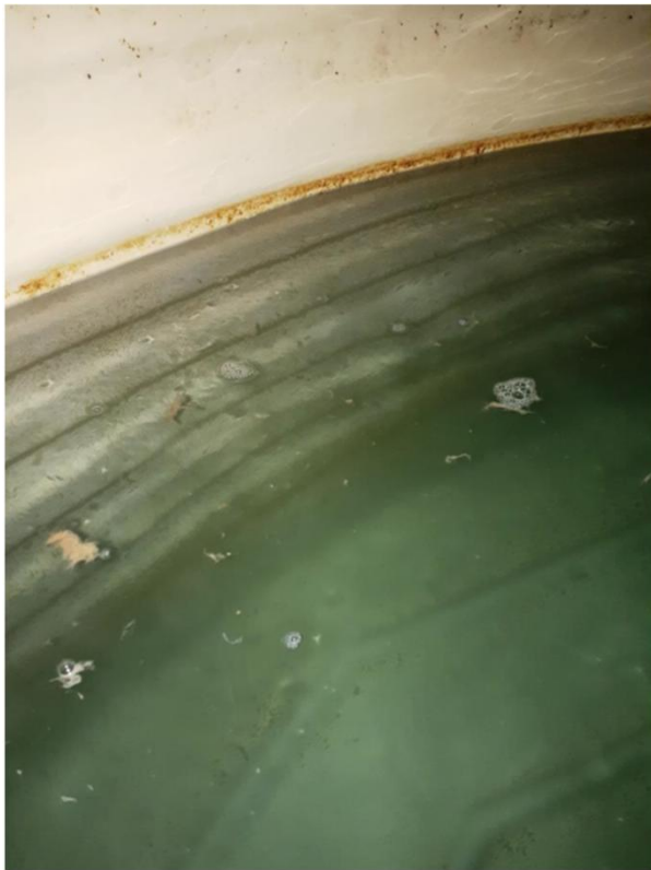
Start of Ultrasonic Test
