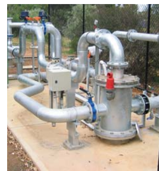
Submersible pump installation
