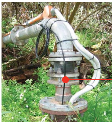
Gunmetal wafer type valve mounted between flanges
