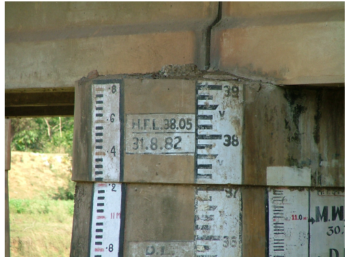
d) High flood level at Nimapara Bridge Gauge Site
