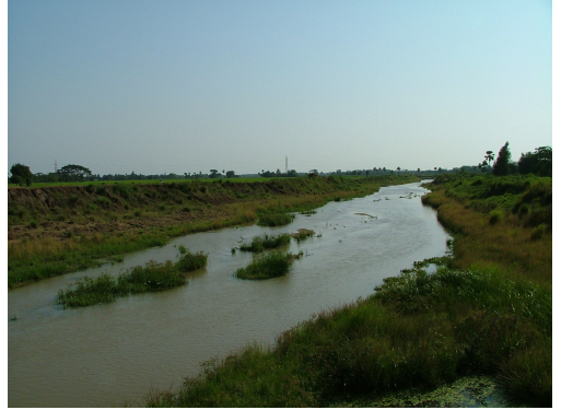
b) Flood Mitigation Canal
