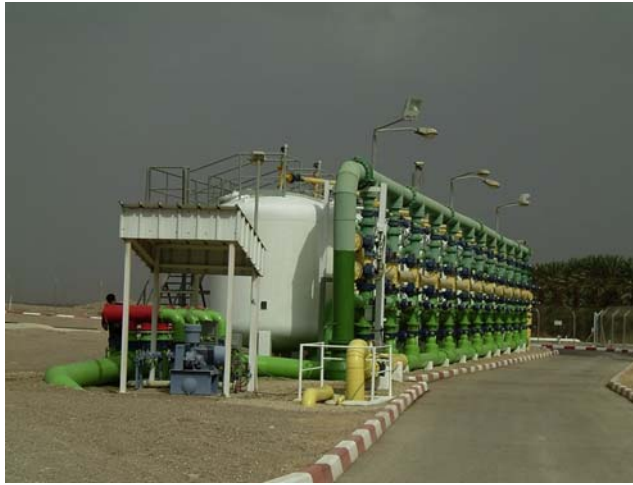
FIGURE 8.6 Vertical pressure filters.
