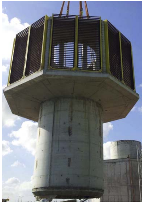
FIGURE 5.1 Vertical intake tower with coarse screen.
