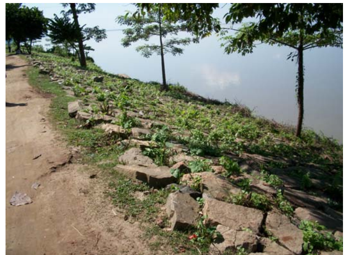
Fig. 12. Existing revetment riverbank protection at Palasbari
