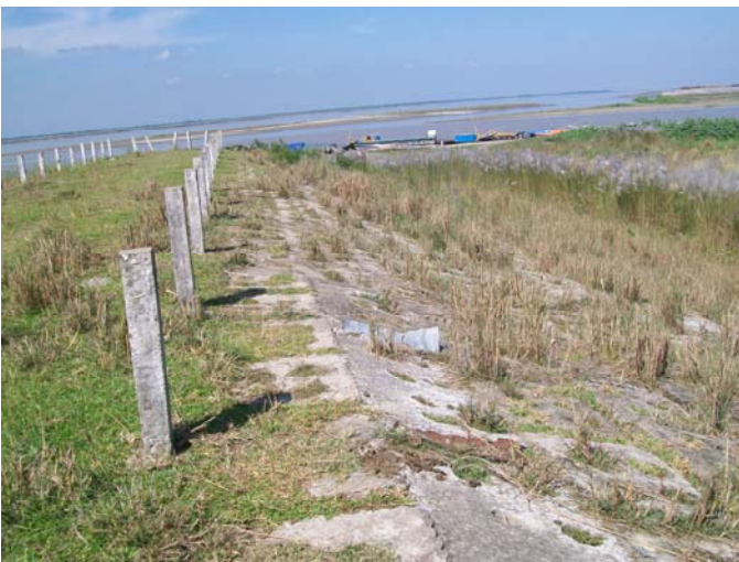
Fig. 3. Views of a typical land spur constructed along the river
