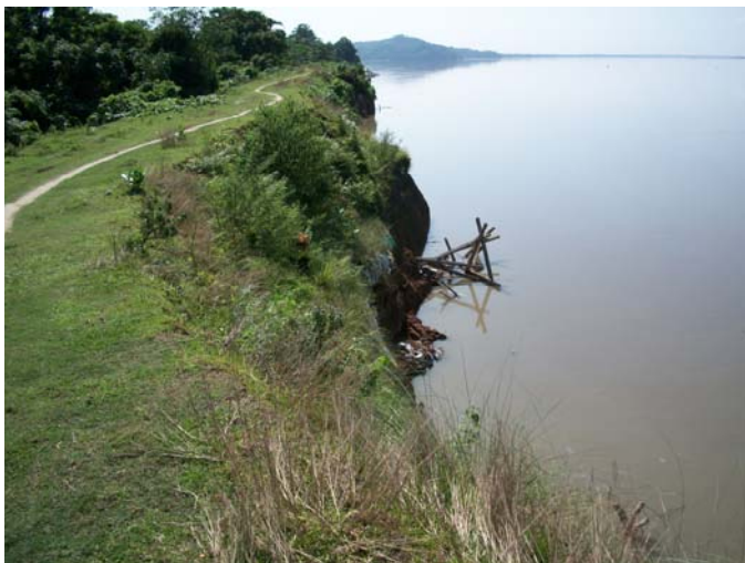
Fig. 11. Some views of riverbank erosion at Palasbari
