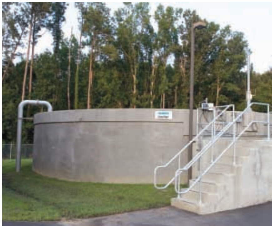
Side-Stream Interchange Bioreactor
